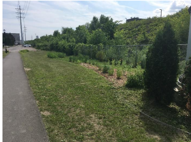
Power line right-of-way between Charland and Fleury substations
