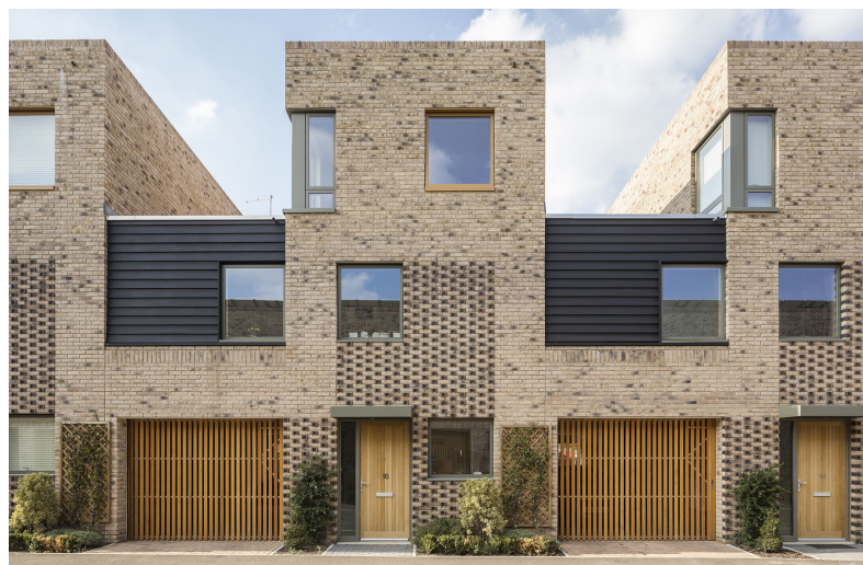
▲ Dissimulation sous les terrasses latérales, Cambridge Housing Community, UK © Proctor and matthews Architects
